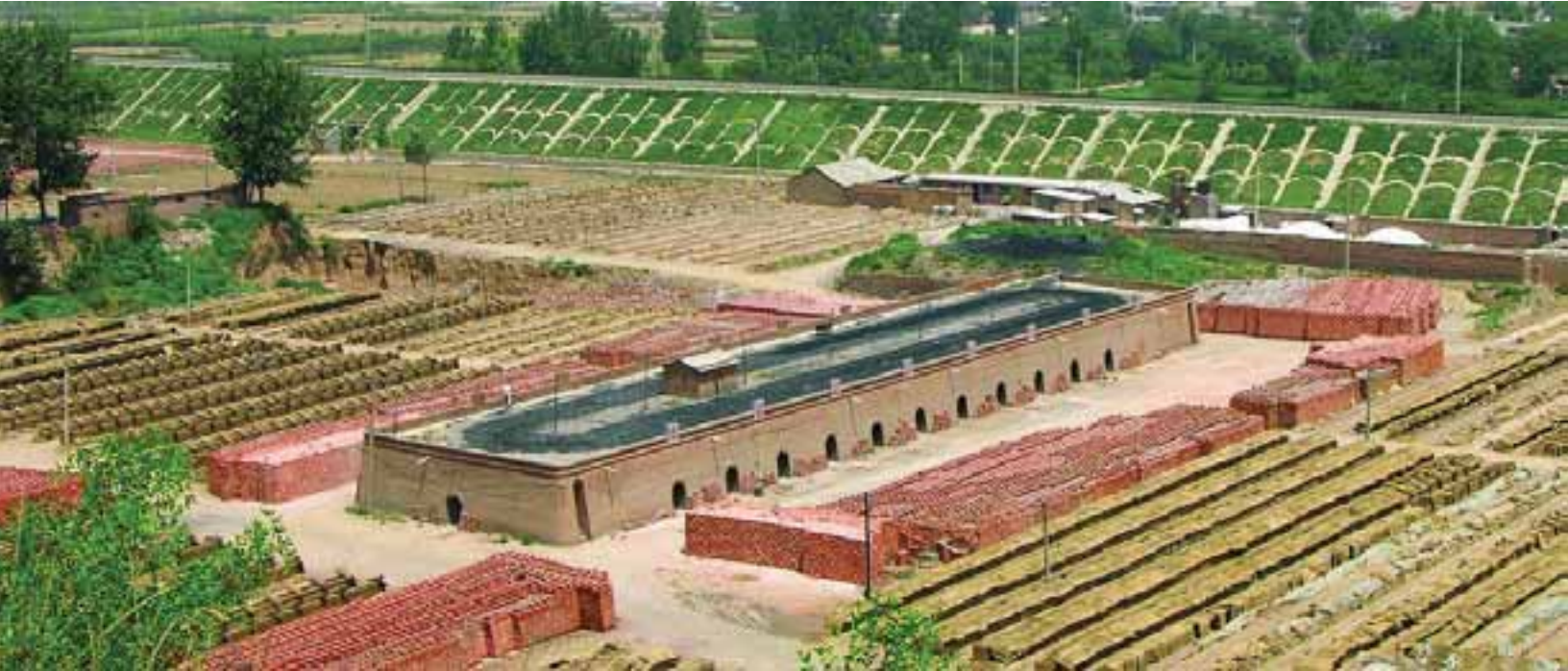
Liucun Hollow Brick Plant, China. GEF supported the construction of this energy-efficient tri-arch brick kiln and promoted the diffusion of this technology in Bangladesh
