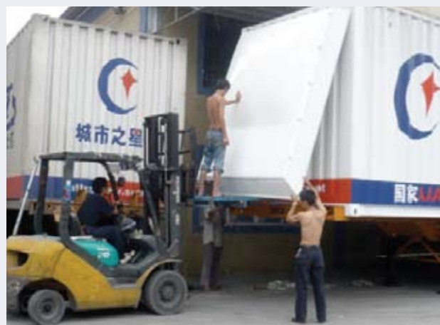
Installing aerodynamic technology Photo credit: World Bank
