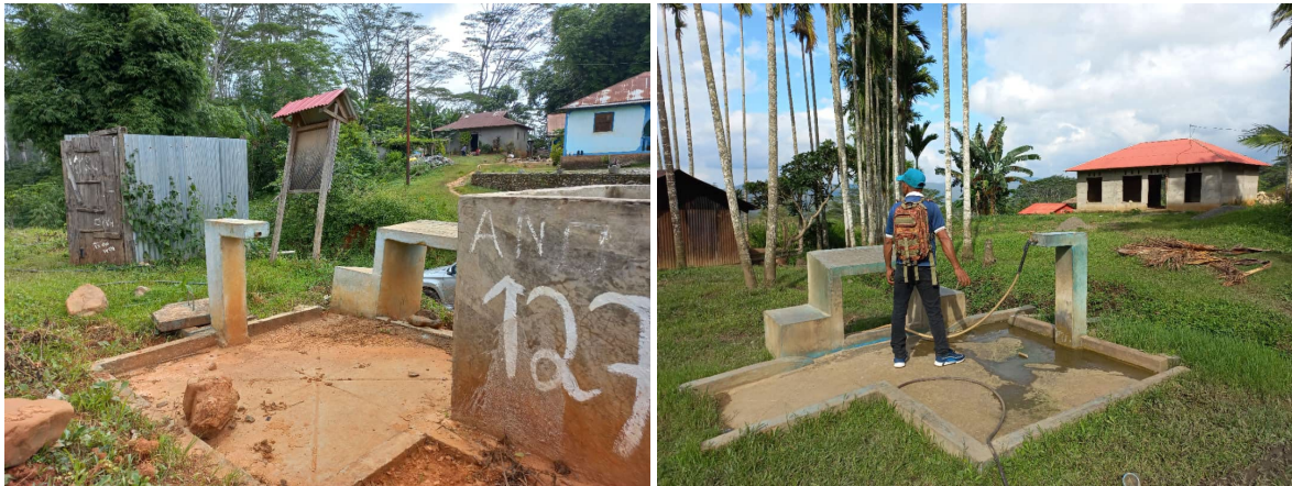
Photo 7: One water collection point that has stopped working (left) and another one that is fully operating near the water source (right) in Talimoro (Ermera)
