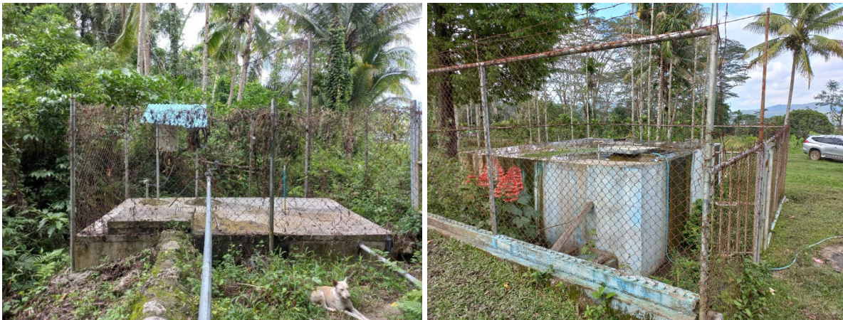
Photo 5: The main water distribution/storage system in Uailili (left) and Talimoro (right) are well-protected. Both systems remain operational to date.
