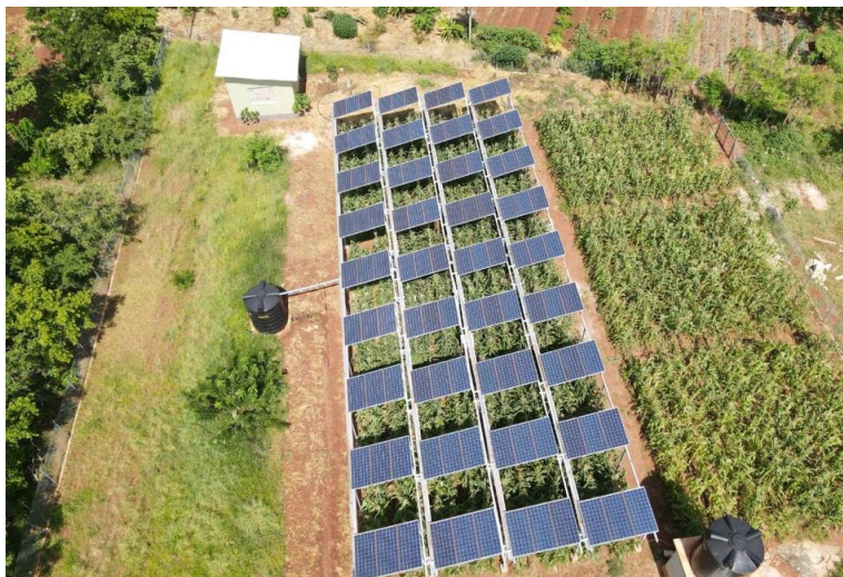
The off-grid AV system used in the Harvesting the Sun Project improved access to electricity, generated higher crop yields, and reduced irrigated water use. Source: Dr Richard Randle-Boggis, University of Sheffield.
