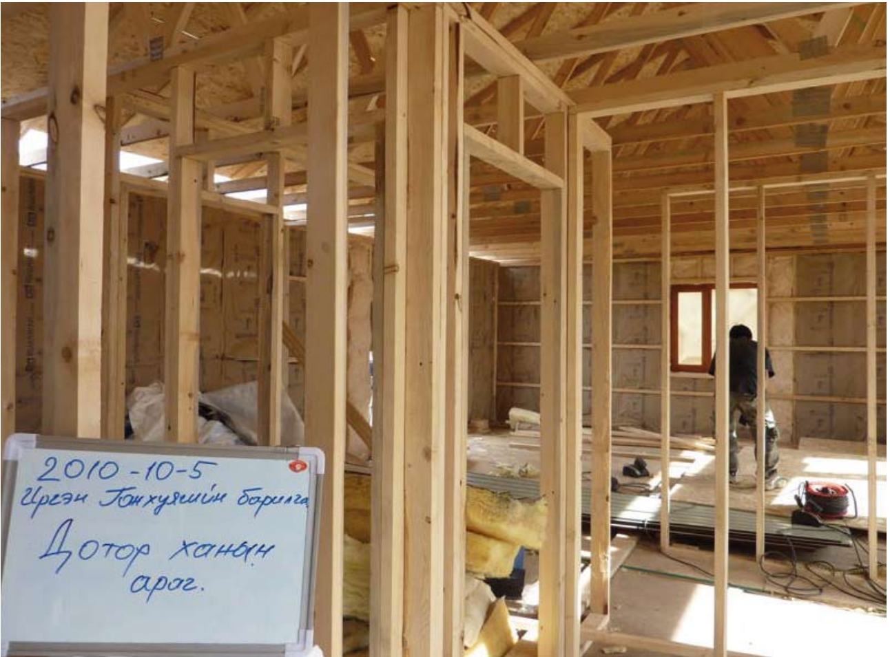
Energy Efficiency Buildings in Mongolia: Timber-frame house construction (inner view) © Ts.Battu
