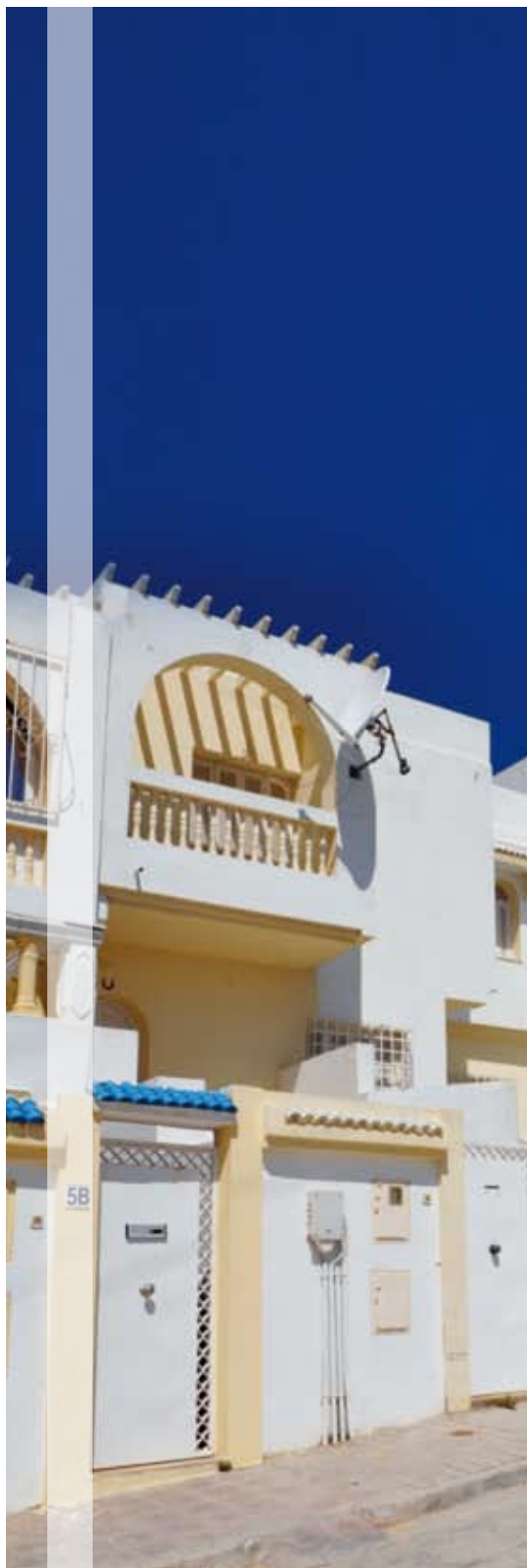
Residential Sector Welfare Housing, Smit. Demonstration projects in Tunisia © Eric Thauvin / AFD
