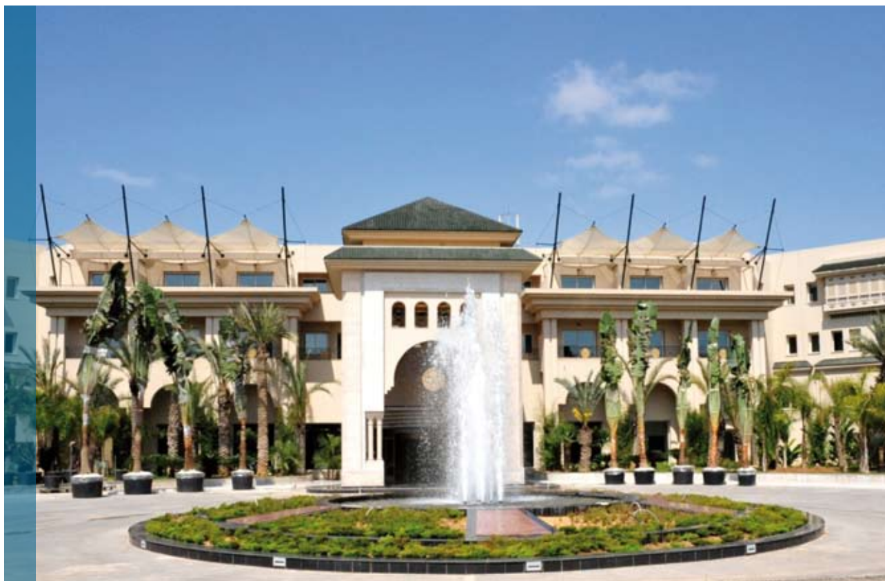
Tertiary Sector Hotel Buildings, Russelior Hotel. Demonstration projects in Tunisia © Eric Thauvin / ADF
