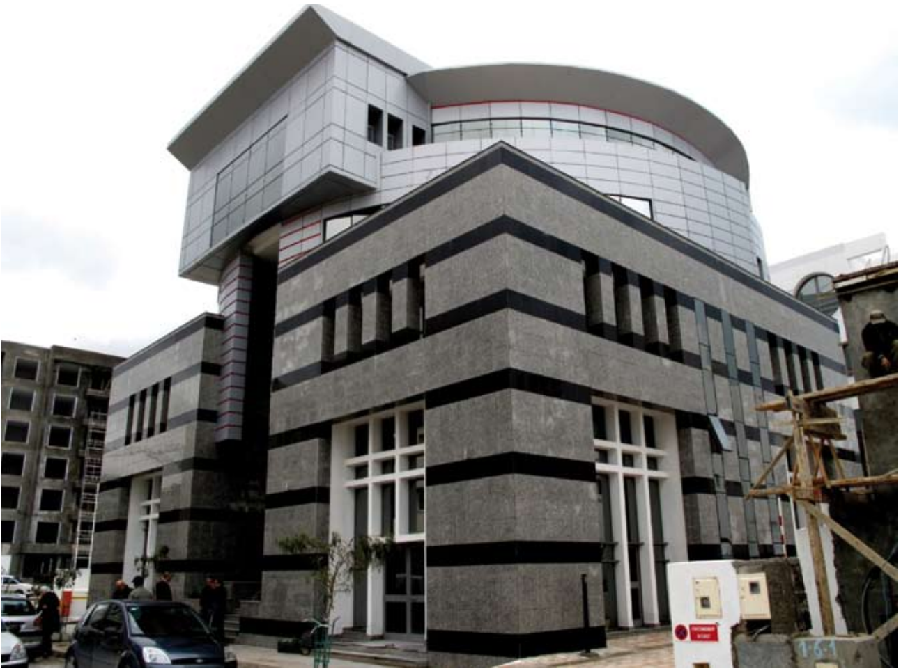
Tertiary Sector Office Buildings, Head Offices of the EPPM Company © Eric Thauvin / ADF
