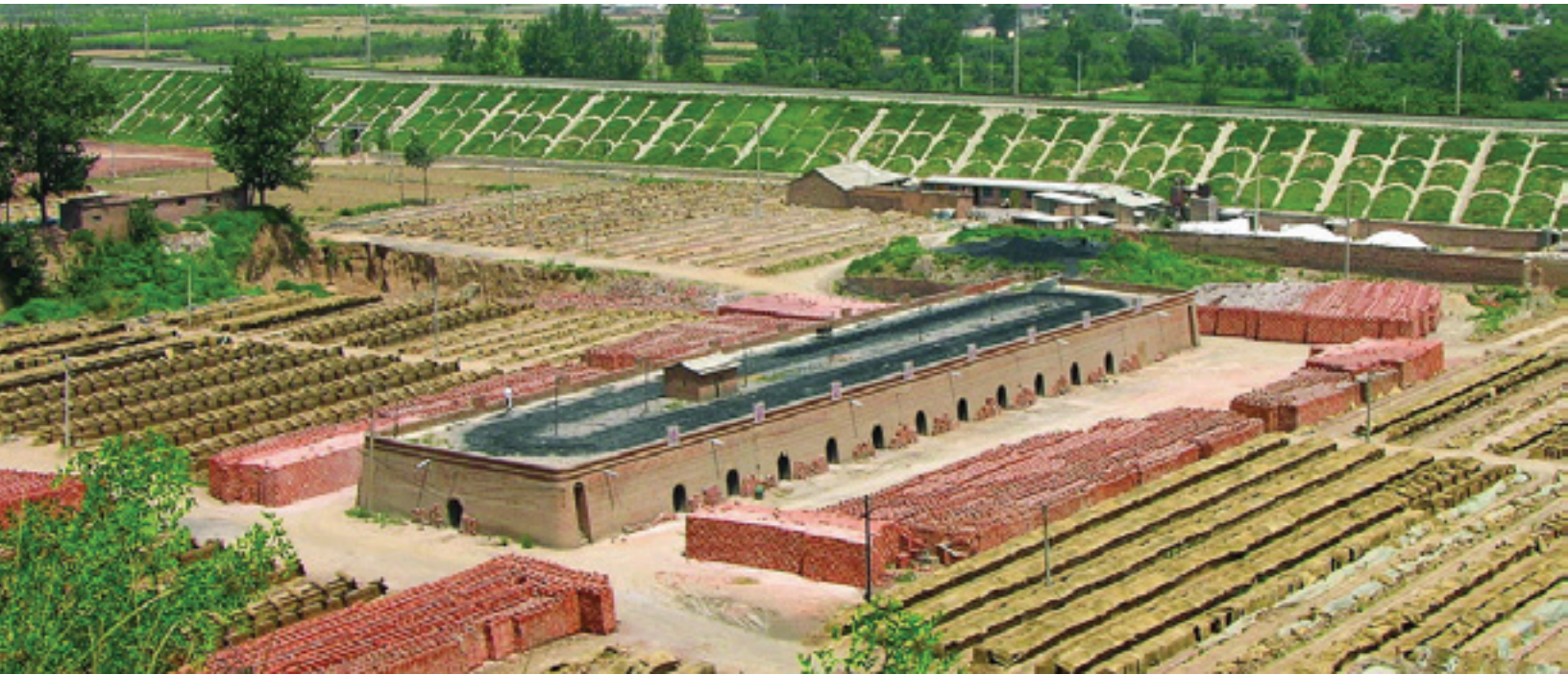
Liucun Hollow Brick Plant, China. The GEF supported construction of this energy-efficient tri-arch brick kiln, and also promoting diffusion of the technology in Bangladesh.
