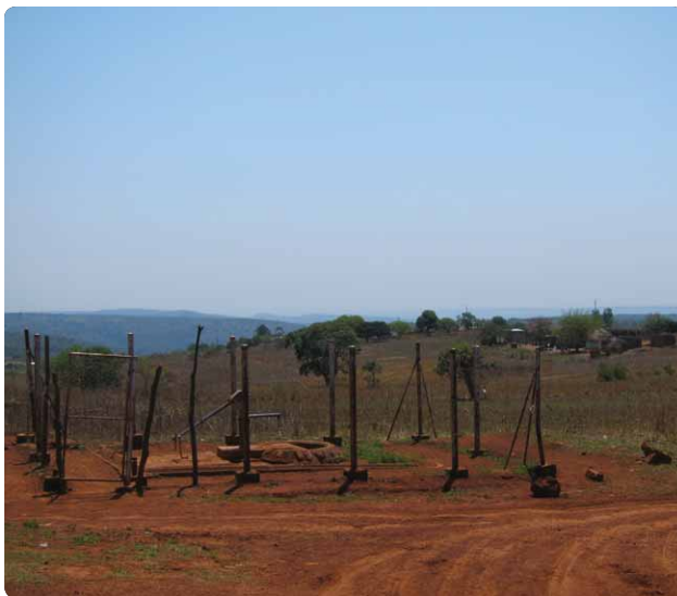
A groundwater pumping station servicing a rural community in the Lebombo Mountains, Swaziland near the Mozambique border / A. Dansie
