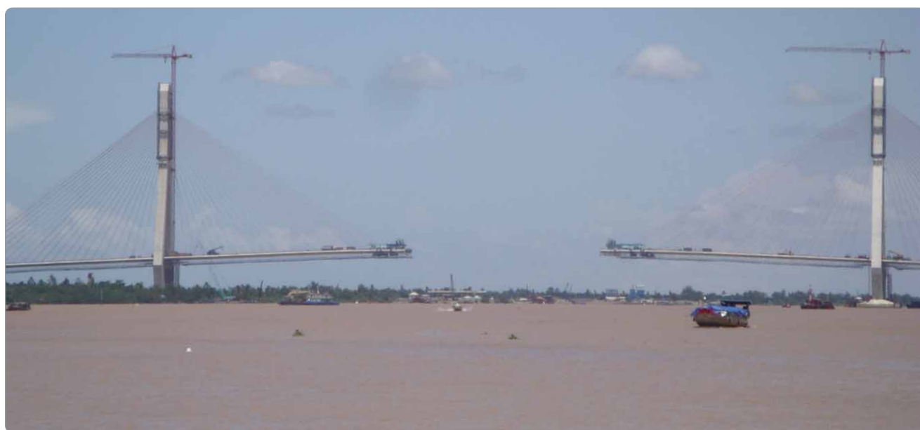
Human population growth in the Mekong Delta is seeing rapid urbanization and land use change, a bridge under construction in Vietnam where ferries were the only option for crossing this part of the delta before / A. Dansie
