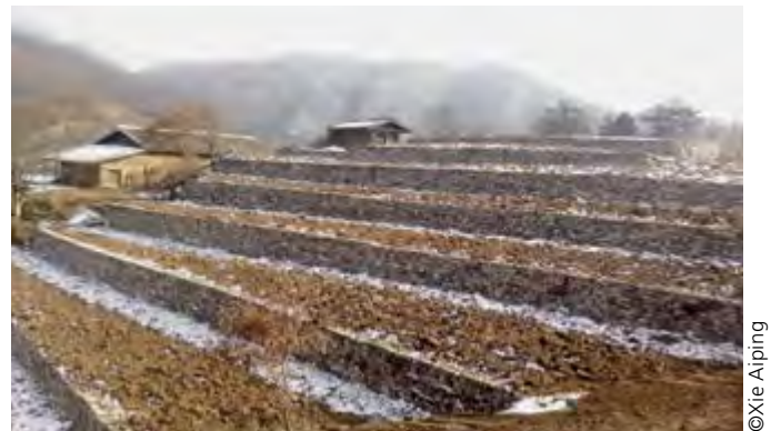
Newly constructed stone dike terraces, Gansu province.
