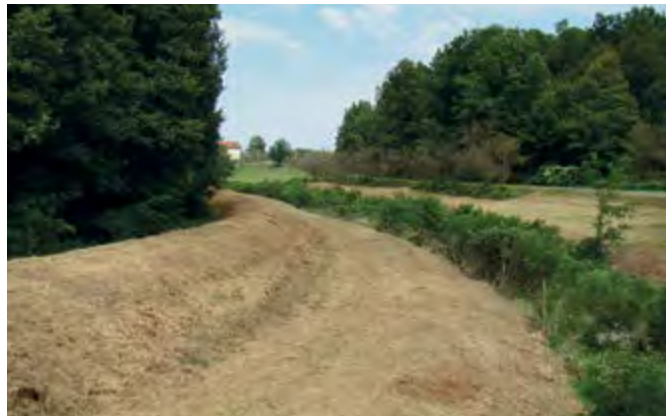
Circumferential (diversion or interception) canals to protect the agricultural area in the plain from mountain waters, Nožičko, Srbac municipality, north Republic of Srpska.
