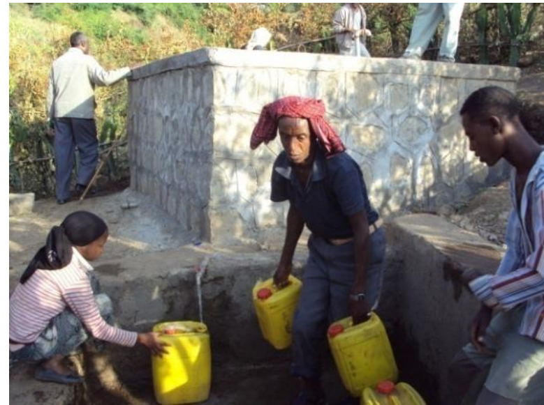
Completed spring development in Kebele, Ethiopia (SCCF)
