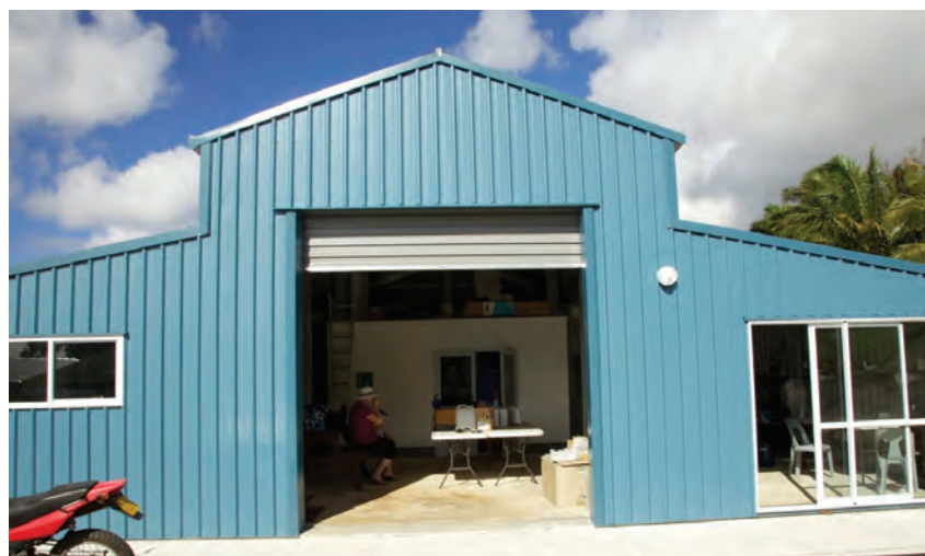
Photo 9. Newly constructed extraction facility on Rarotonga for the CIMTECH Technology. Photo Lorinda Matheson.
