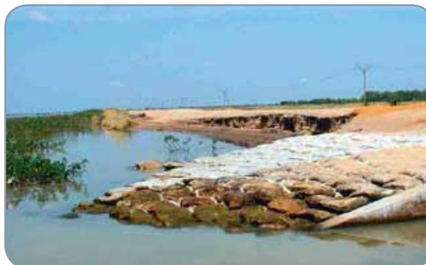
Erosion and Sand Bag Protection on the Inside Dam Wall of the Maga Dam (south of Lake Chad) (Lake Chad Basin GEF project).
